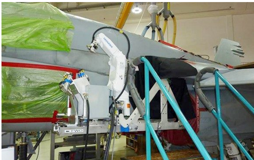
Figure 28 Blending of two critical locations on Former 395 with the help of a robot
