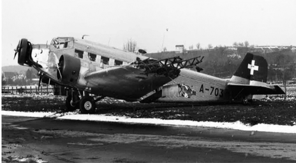
Figure 16 Serious damaged left wing HB-HOP after a crash on the ground (1965)
