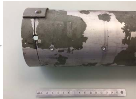
Figure 10 Crack on the disassembled spar
