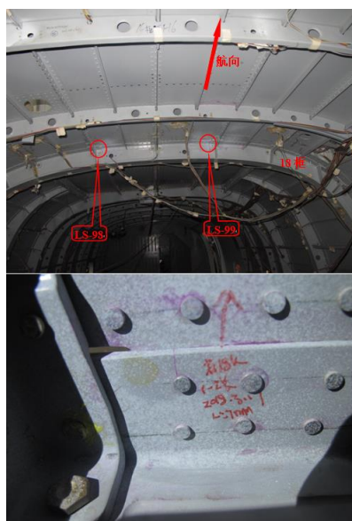
Figure 6-18 Crack at the rivet hole in spar
